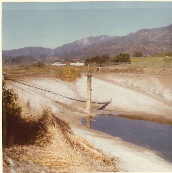
Outlet tower and culvert Spillway in background
