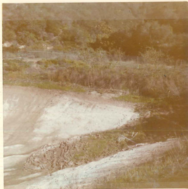
Embankment failure main canyon into reservoir
