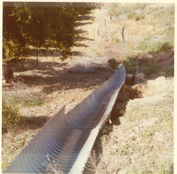
Erosion under left abutment ditch
