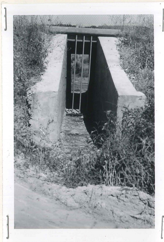
Picture looking upstream through spillway showing grill over exit portal.
