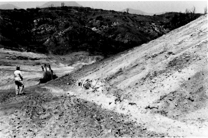
Closeup of sandy soil along left abutment which was later partly removed. (See Report).
