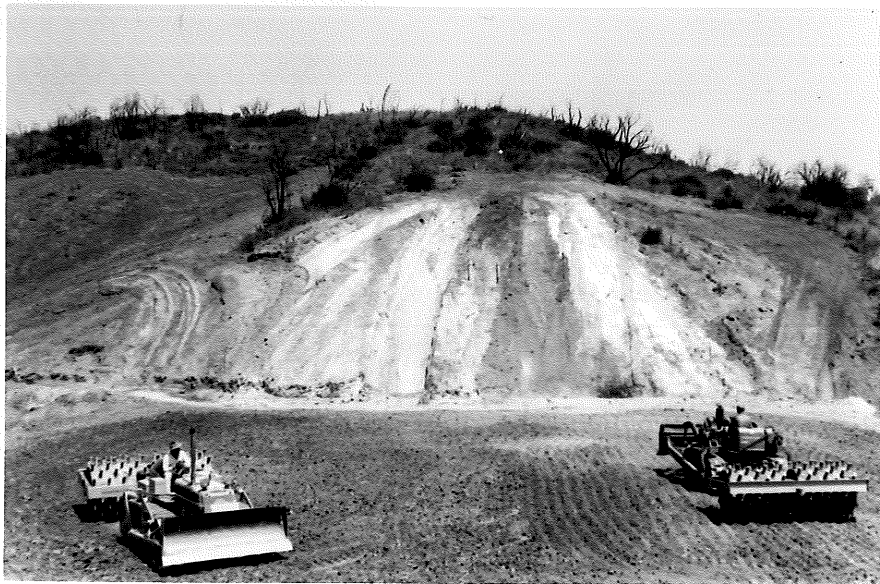
Looking towards left abutment which is very soft sandstone which breaks down easily and forms a pervious sandy zone along abutment.
