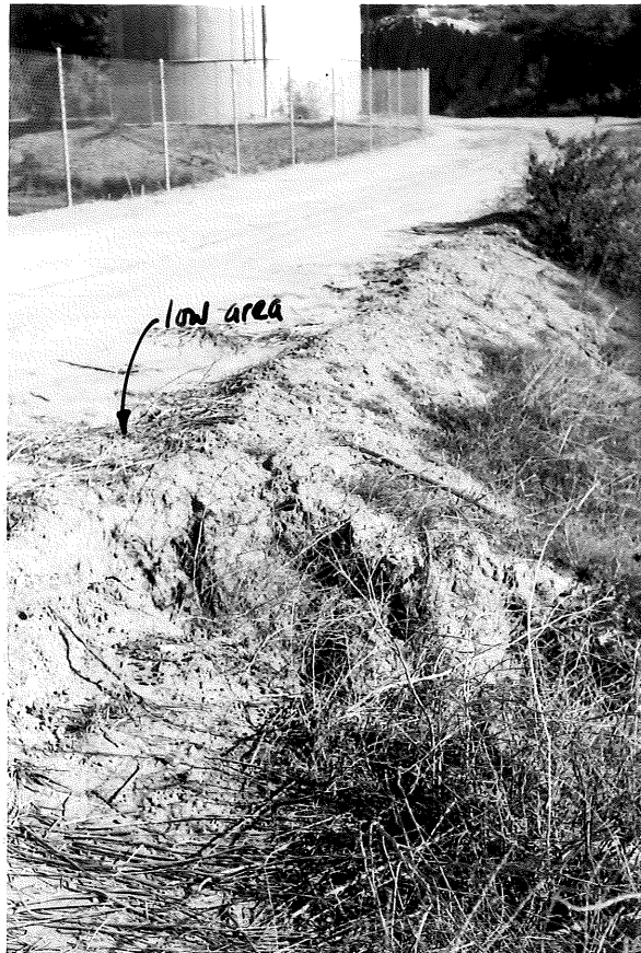
View shows area of low spot in crest and erosion gully on the downstream slope.
