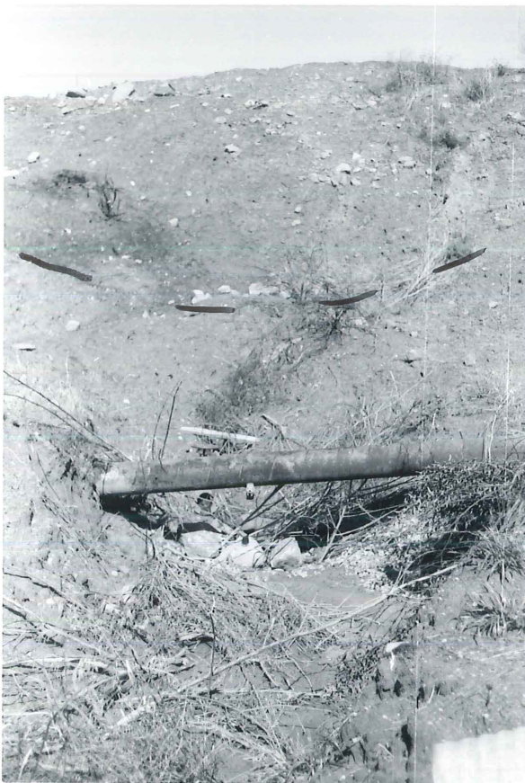
View of small shallow slide along the northerly edge of the reservoir.
