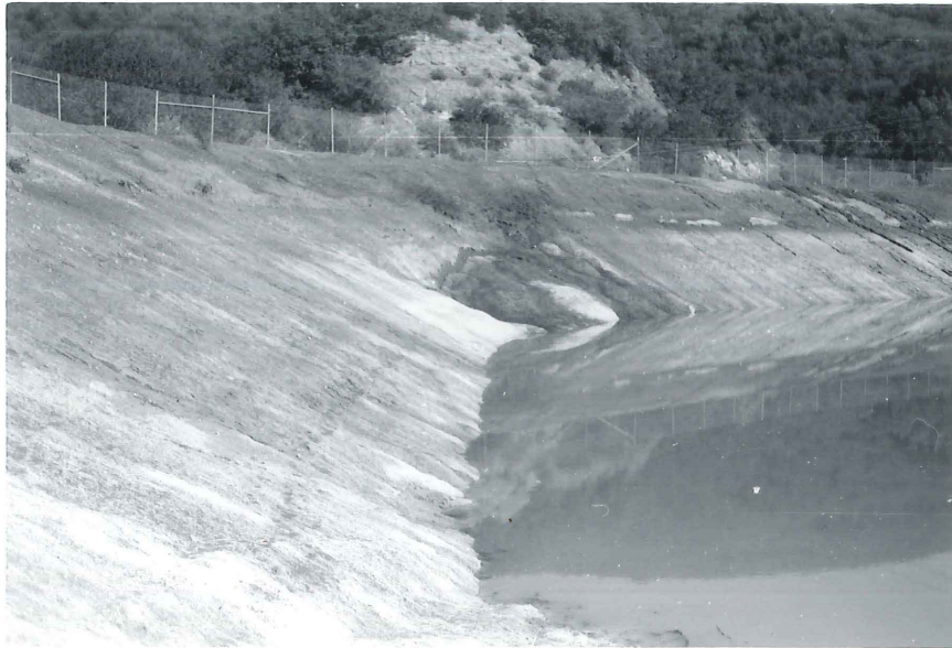
View of small shallow slide along the northerly edge of the reservoir.
