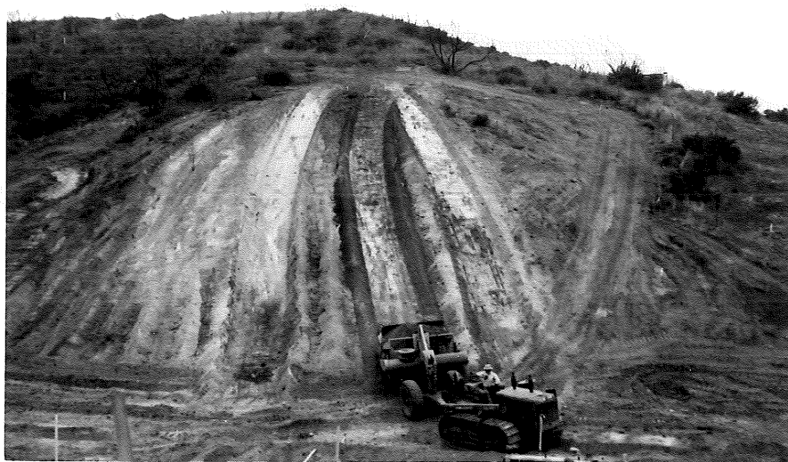
View of left abutment showing light soil cover over soft sandstone.
