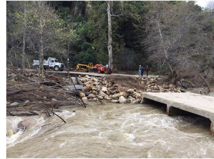
Spring 2018 - embankment repairs after washout
