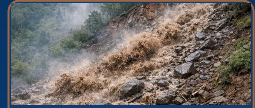
04 Landslide / Debris Flow
