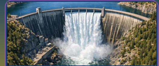
08 Dam / Levee Failure
